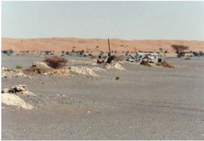
Line of access shafts to a dawoodi falaj in Wadi al Batha, Oman. Photo by Sue Hutton .
