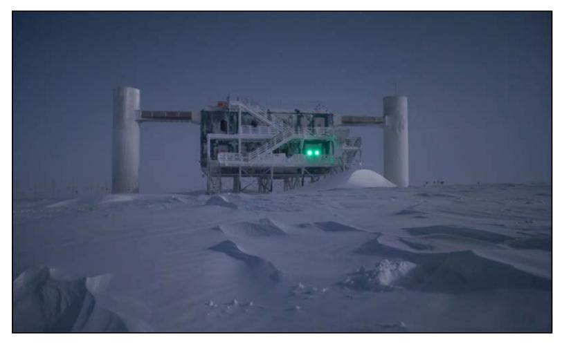
This is the <u>IceCube Neutrino Observatory</u> in Antarctica. Actually most of it is deep under the ice. Almost 90 wires, each with 60 detectors attached, were lowered into holes melted in the ice using a hot water drill. And recently they've found some neutrinos with astoundingly high energies — up to 1 PeV!
